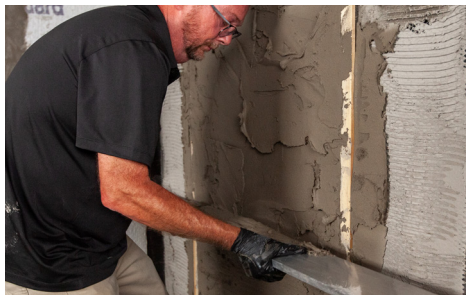
Nonsagging/nonslumping – easily screedable on walls
