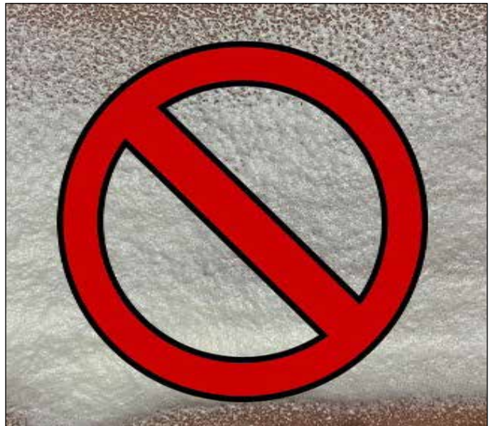
Image 2: Improper adhesive application
