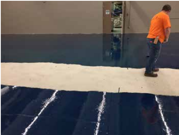
Figure 3. LiquiDam™ being installed
