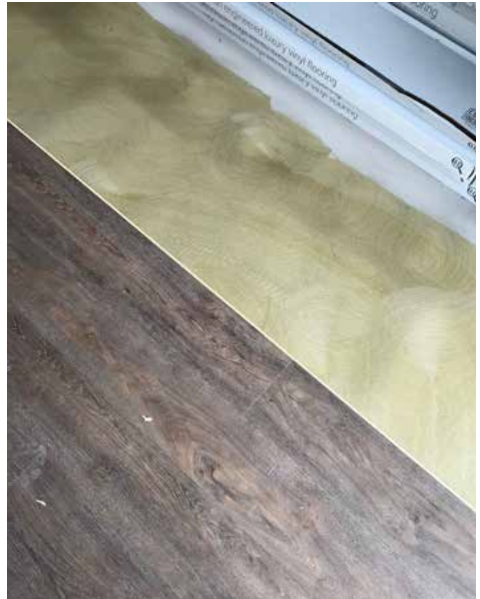
Figure 2. TrowelFast™ being used to install luxury vinyl plank
