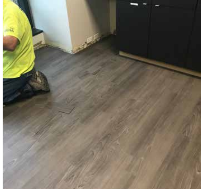
Figure 4. Luxury vinyl plank installation in a break room needed to be able to accommodate foot traffic by lunch time. Flexera allowed this quick turnaround.
