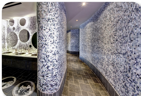
Glass tile / non sag for walls
