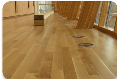
Fast cure allows for efficient installations
