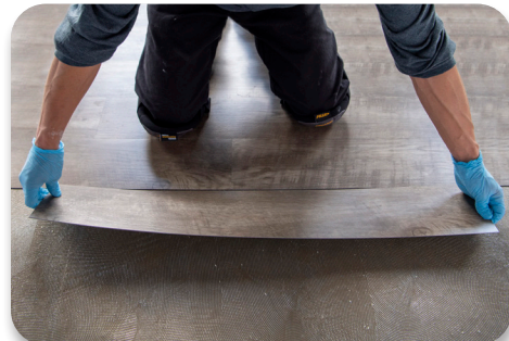
Immediate foot traffic after PSA method installation
