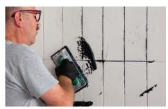
Pigment particles are integrated within the grout making installation and clean-up fast and easy
