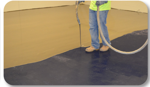
No priming required prior to installation of SLUs
