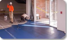
Eliminate labor for mixing – just trowel and back roll or roll-apply
