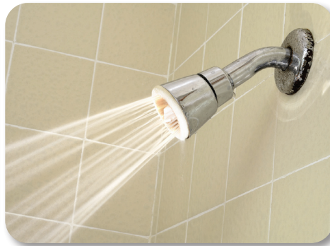
Open to water exposure in 72 hours
