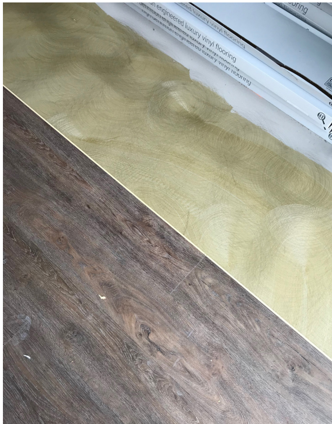
Figure 2. TrowelFast™ being used to install luxury vinyl plank
