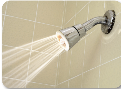
Open to water exposure in 72 hours
