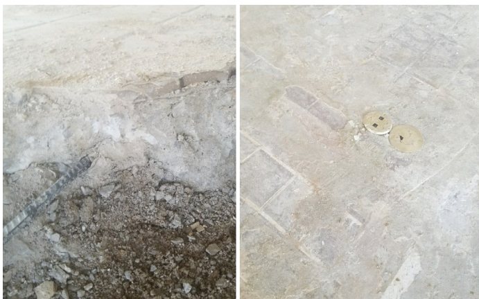
The flooring prior to renovation.
