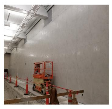
The tile panels were then grouted with TEC Power Grout® Ultimate Performance Grout. Well-known for its stain and water resistance, Power Grout was selected to handle the challenges it would certainly face in the natatorium. Additionally, TEC Fast Set Deep Patch and TEC AccuColor 100® 100% Silicone Sealant were used throughout the project for filling the voids and joints and at transitions between the materials.
