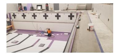
For the pool tank and gutter, the installation team opted for the following products: TEC® Fast Set Deep Patch, TEC Floor Mud and TEC Xtra Flex™ Acrylic Latex Additive for prepping the tank. For waterproofing, the team used TEC HydraFlex™ Waterproofing Crack Isolation Membrane.
