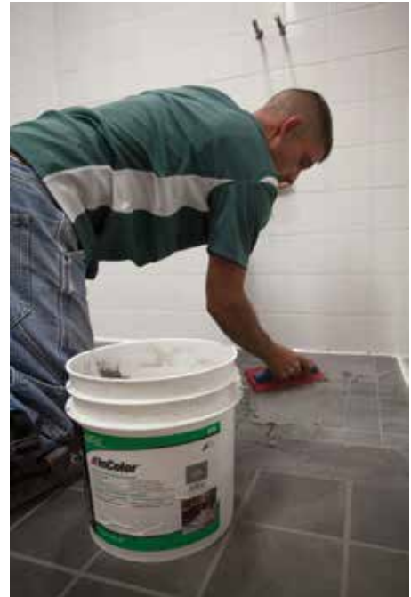
TEC® InColor™ Advanced Performance Grout, in Light Pewter, Bright White, Light Smoke and DeLorean Gray, was used with all of the many tile types in the North End Zone Complex.
