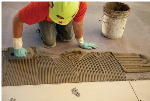
The best mortars for exterior installations combine bond strength with flexibility to allow for shifts in the substrate caused by changing moisture and temperature levels.
