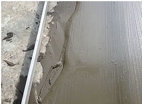
A patching compound, like TEC® Fast-Set Deep Patch , can be used to address substrate variation.
