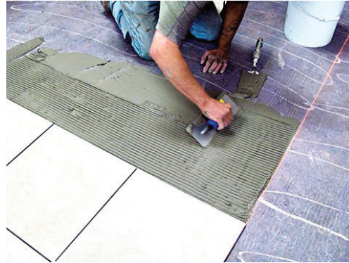
The tile is bonded directly to a waterproofing and crack-isolation membrane.
