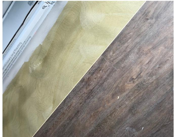
**Figure 2.** TrowelFast™ being used to install luxury vinyl plank
