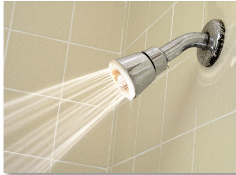
Open to water exposure in 72 hours
