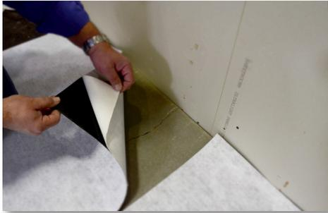
Easy to install – just peel off the backing, then press into place on the primed surface.
